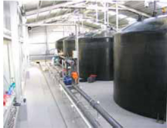
PacifiCorp (Moab, Utah) 2MWh VRB-ESS (VRB Power Systems)
