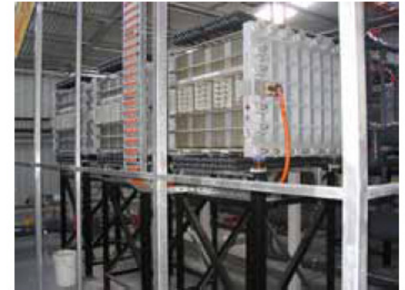
PacifiCorp (Moab, Utah) 2MWh VRB-ESS (VRB Power Systems)
